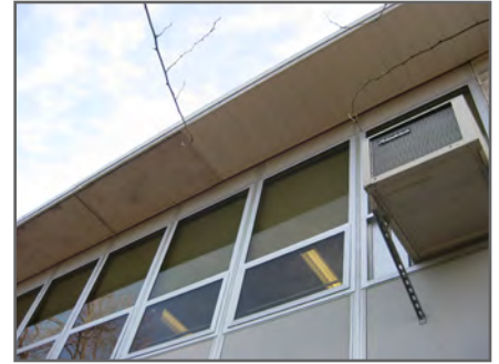
Missing soffit panels should be installed.
