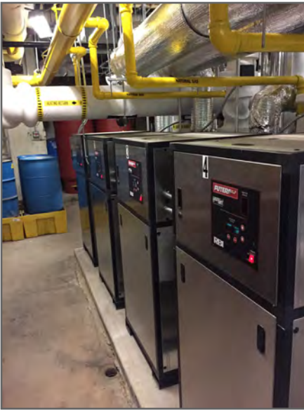
New Boiler Plant
