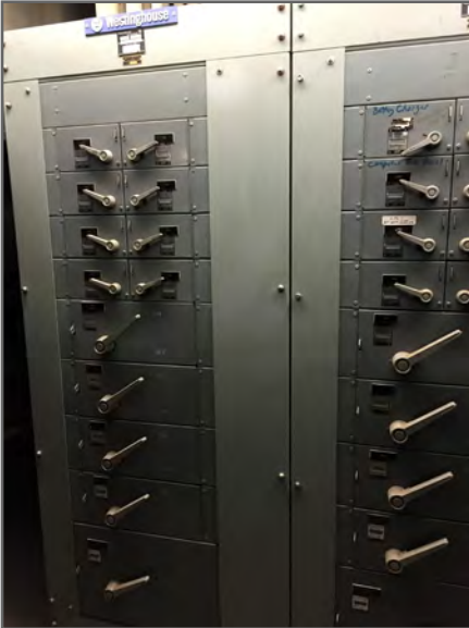
Main Electrical Distribution Equipment
