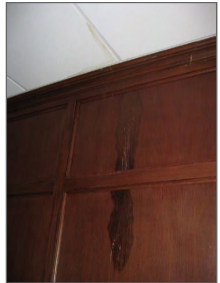
There is evidence of several roof leaks in fifth floor offices.
