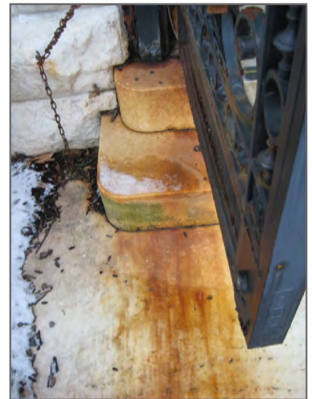
Many of the ornate, metal doors are rusted
