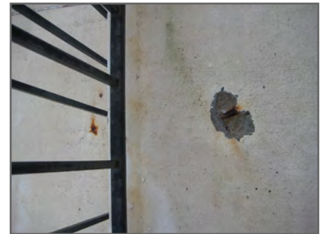
The exterior concrete ramp is spalling
