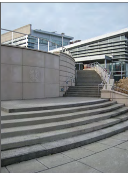
The site stair should be repaired.
