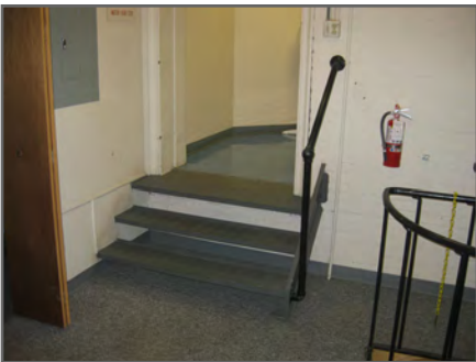
There is no accessible route to the large conference room on the second floor.
