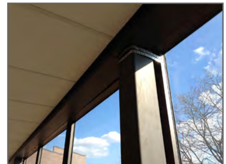
The failed curtainwall on the third floor has to be strapped to the building structure.
