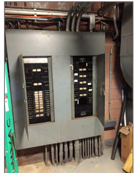
Existing electrical distribution equipment is nearing the end of its useful life.
