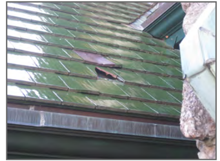
Damaged roof tiles should be replaced.
