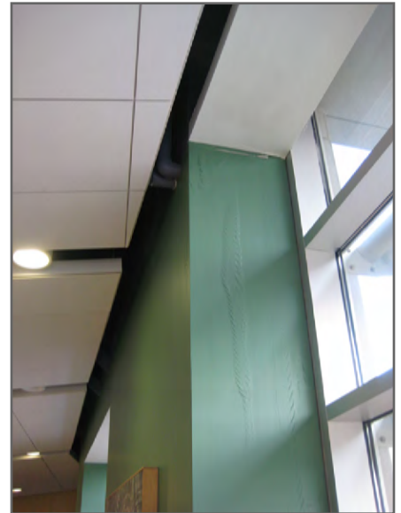
There is evidence of a leak in the second floor corridor adjacent to the Learning Center.
