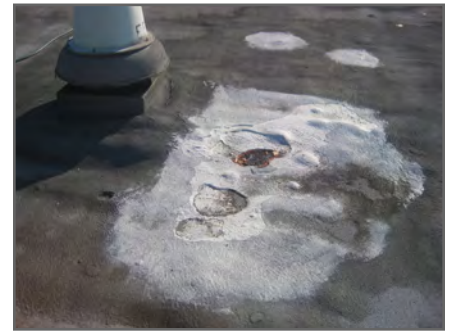
The roof should be recoated or replaced.
