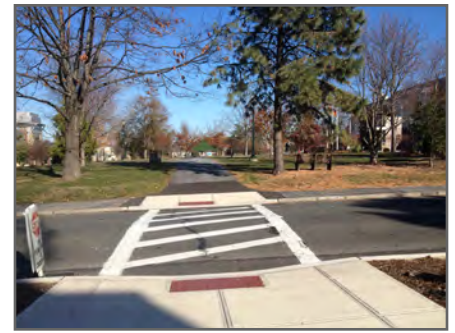
Improved crosswalks with accessible curb ramps have recently been installed at this crossing. All crossings on campus should be brought to this level of accessibility.
