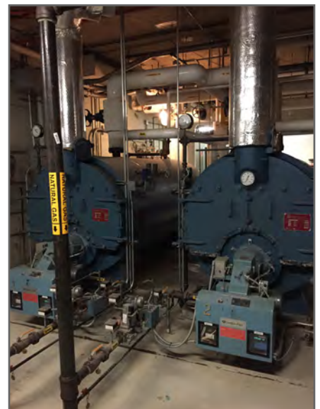
Existing Harriman Hall Boilers
