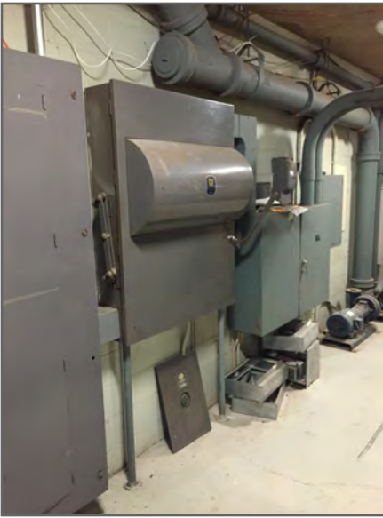
Existing Electrical Distribution Equipment
