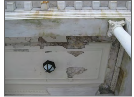
Exterior plaster ceilings are in poor condition
