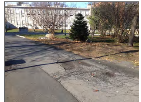
Pavement condition was identified as poor if there was significant cracking and spalling that pose a safety hazard.
