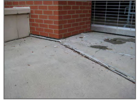
Sealant between the building and sidewalk has detached in some areas.
