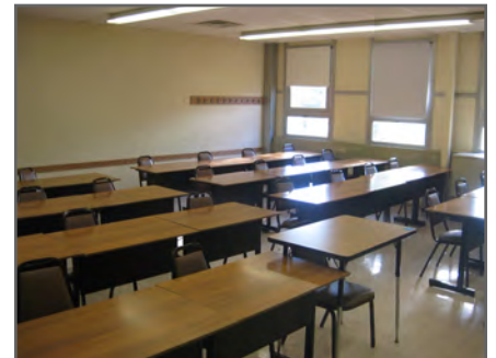
Interior finishes should be replaced to improve the appearance of the building.
