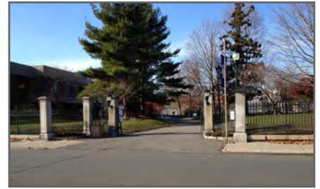
Continuing the concrete sidewalk across the main campus entrance would help establish the hierarchy of pedestrians first.
