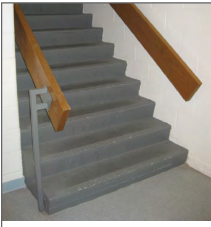
Existing handrails should be replaced with fully-compliant handrails.
