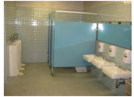
Toilet rooms require additional modifications to bring them into full compliance.
