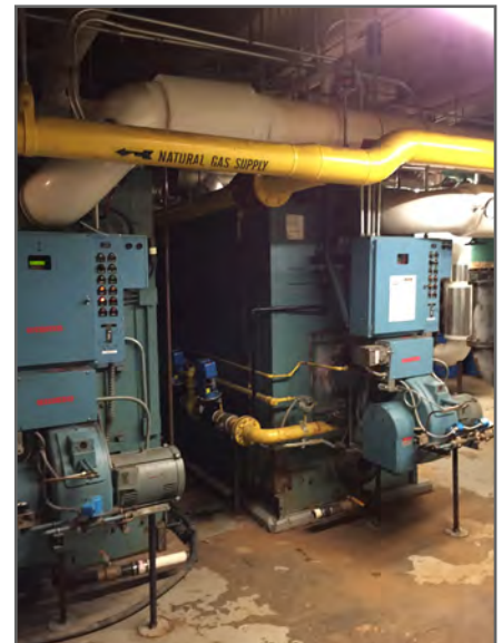
Existing Boiler Plant
