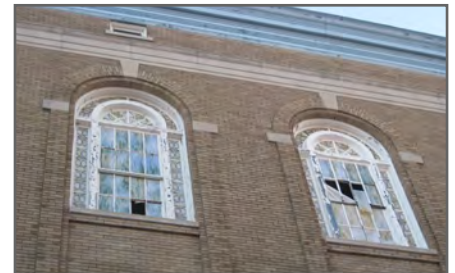
Damaged windows should be replaced.
