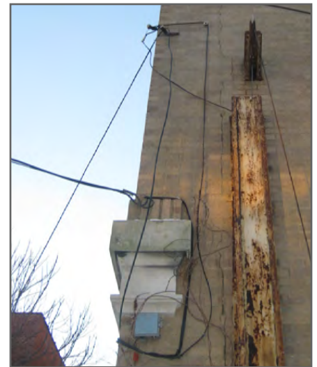
Cracks on the southeast corner may indicate building settlement.
