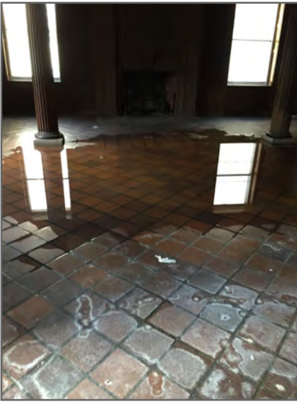
At the time of the site visit, there were large puddles of water throughout the building.
