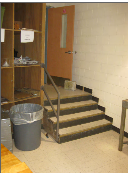
Art Classrooms 113 and 115 have stairs at the entrance door and are only accessible by traveling through Art Classroom 117.
