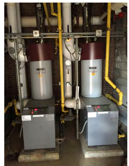
Recently Replaced Boiler Plant
