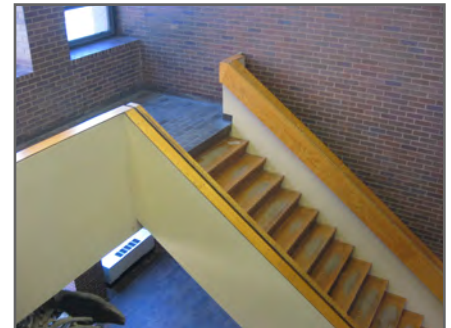
The guardrail at the open stair is less than the code required height.
