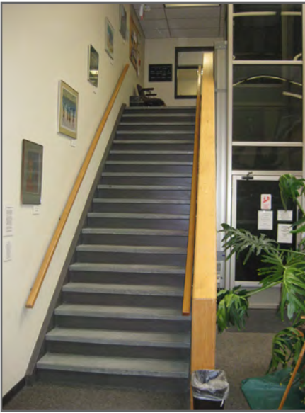
Existing handrails should be replaced with fully-compliant handrails.
