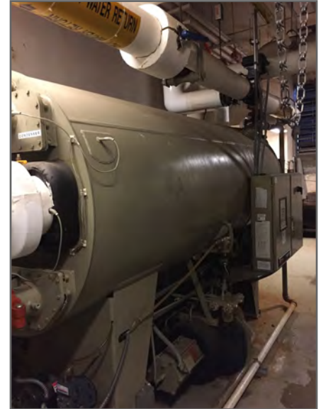
Existing HVAC Equipment
