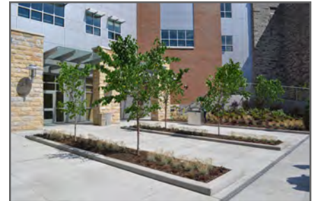
Storm water planters, such as the recently installed ones at the Rowley Center, will be more commonplace as runoff reduction becomes more important.
