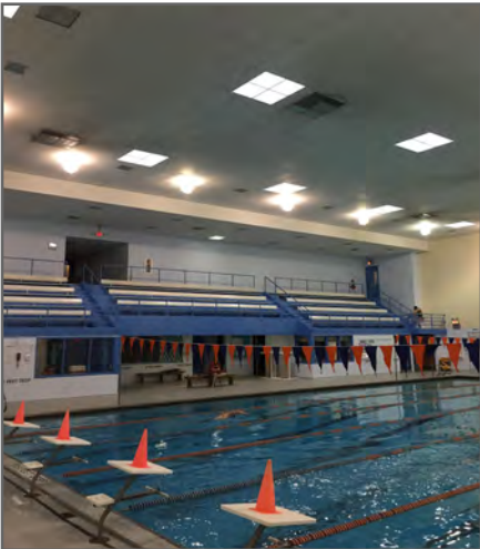
Existing lighting in the pool area should be replaced.
