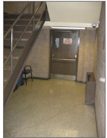
A cane detection railing is required where the vertical clearance is less than 80 inches.
