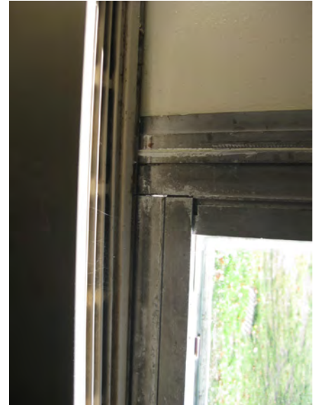
The exterior curtainwall system is poorly insulated and in poor condition.
