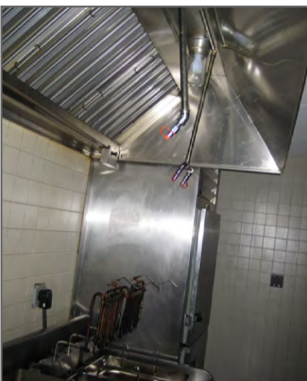
Fire code issues and maintenance concerns prevent use of the grill in the kitchen.
