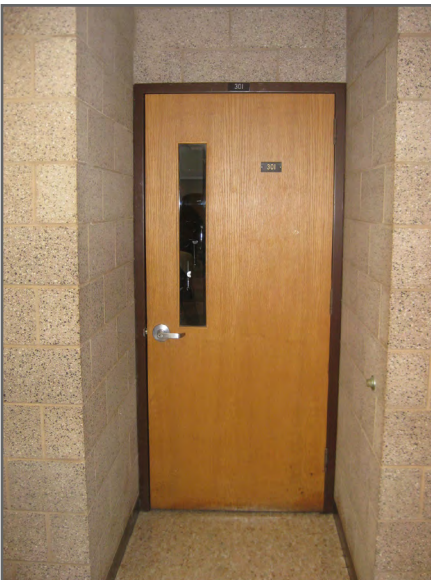
Recessed corridor doors do not have the required clear space at the latch side of the door.
