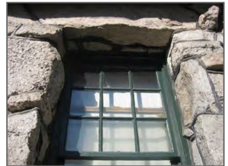
Double-glazed, energy-efficient windows should be installed.
