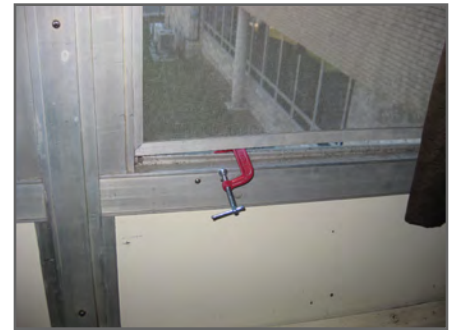
The curtainwall system is in poor condition and, in some places, being held together with clamps.
