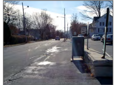
Continuing the concrete sidewalk and curbing north from the Morrison Lab School across Parking Lot #11 driveways will increase pedestrian safety.
