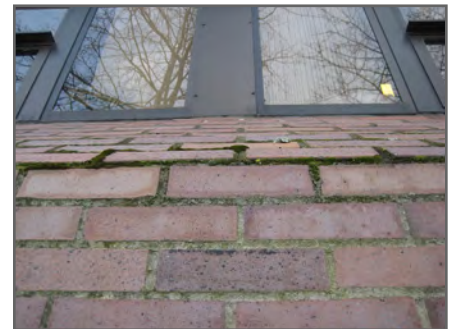
Mortar joints at sloped walls beneath windows are in poor condition.
