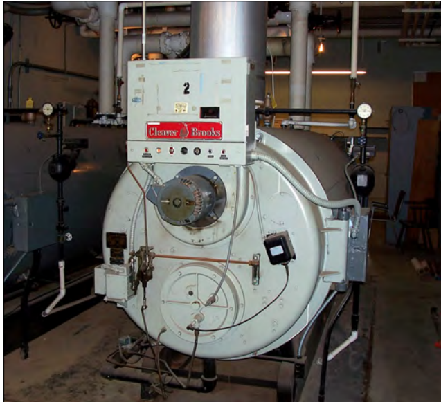
The original boilers are past their useful life and should be replaced within the next ten years.
