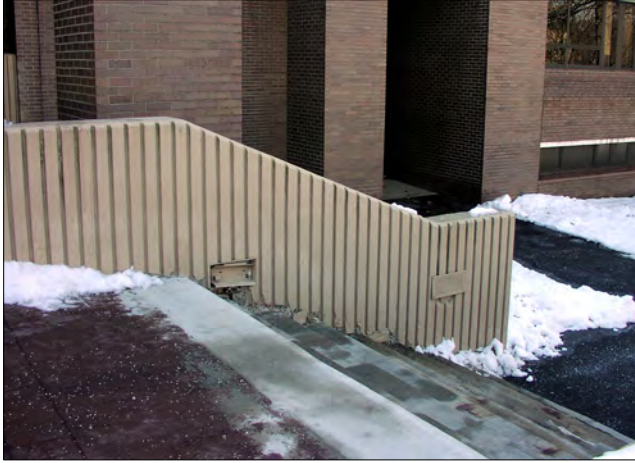
Damaged site stair lighting fixtures should be replaced.
