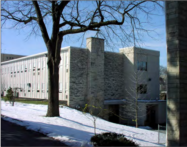
The new elevator addition can be seen at the right of the photo. Small study spaces were created on the second and third floors in the elevator lobby area.
