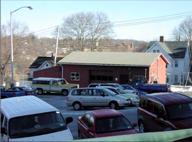
The HVAC Shop sits behind Horton Hall.
