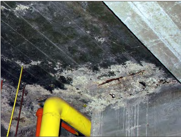
Water infiltration in basement below the ramp is resulting in deterioration of the concrete structure.
