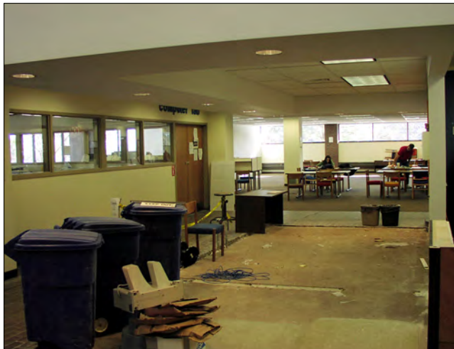
Renovations are underway on the first floor. This is a view past the new circulation desk on the right into the future Information Commons.
