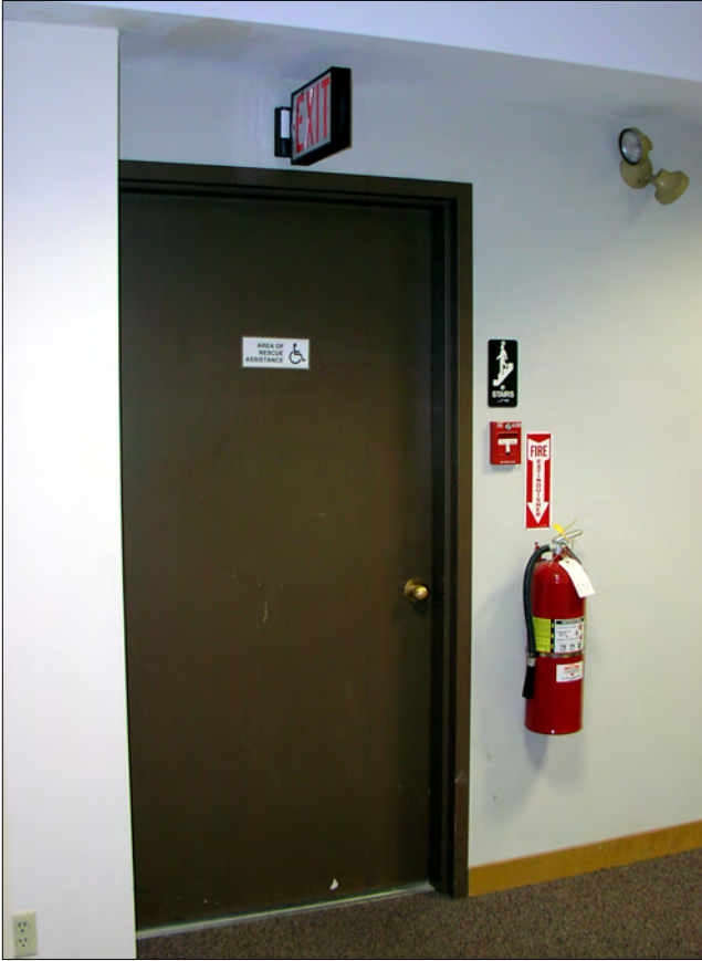
Lever door hardware should be installed at all exit stair doors.
