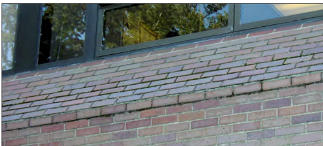
Deteriorating mortar joints should be raked and repointed to prevent further damage to the wall system.
