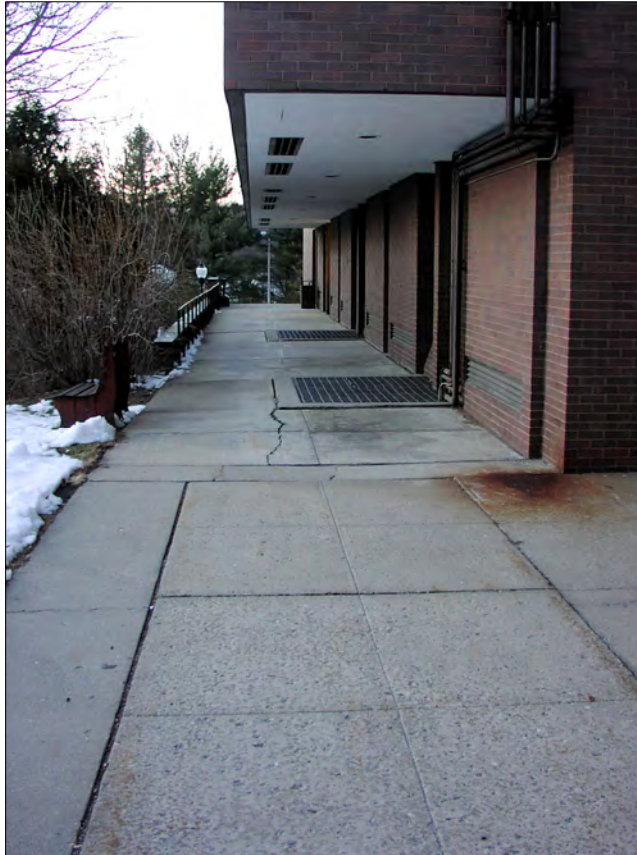
The sidewalk northwest of the Bio-Tech Building is in poor condition and should be replaced.
