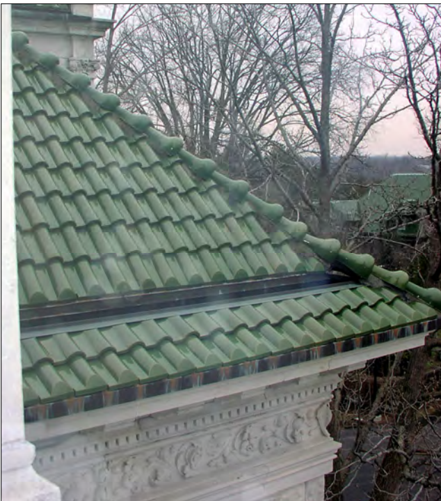
Gutters originally used steam to help melt snow and ice on the roof. This system was not duplicated when the new clay roof was installed.
