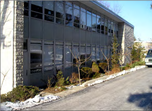
An access ramp is needed at Sarah Wells to make at least the quad level floor accessible.
