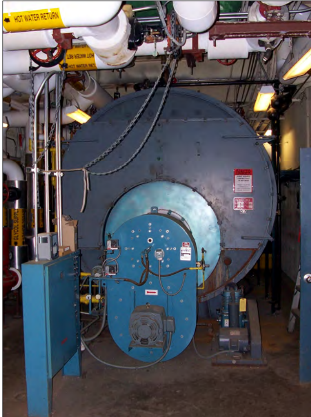
A small boiler should be installed for summer use so the large 600-Hp boiler shown above does not have to be used during summer months.
