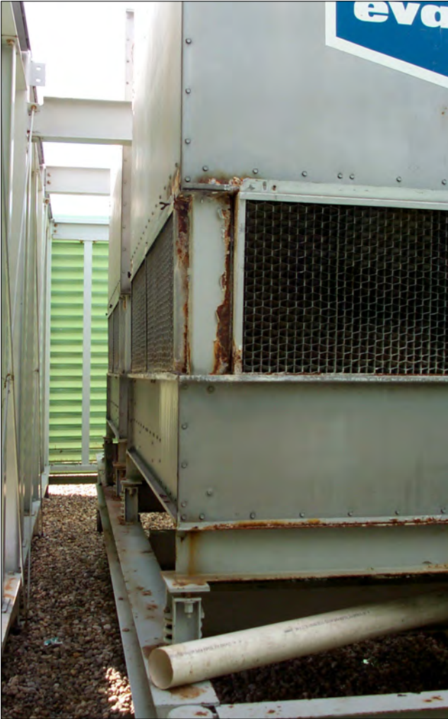
The two open cooling towers should be replaced.
