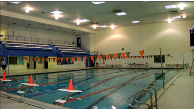
The suspended ceiling above the pool should be removed and the lighting fixtures should be replaced.
