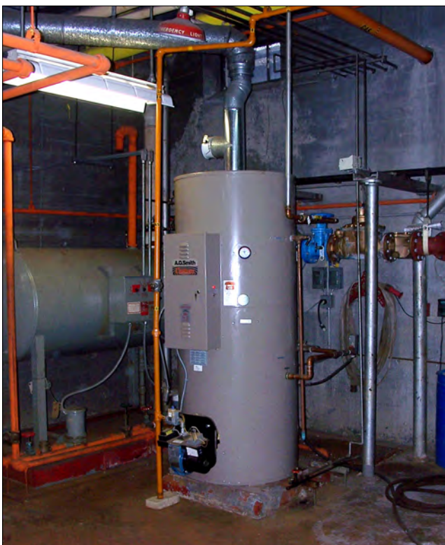
A new natural gas-fired domestic water heater was installed in 2001.
