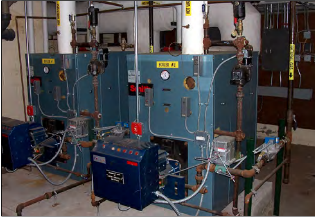
New boilers were recently installed.
