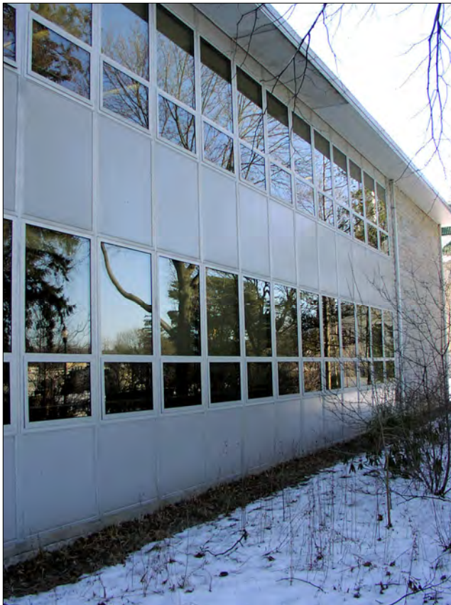
New windows were installed to improve energy efficiency and occupant comfort.
