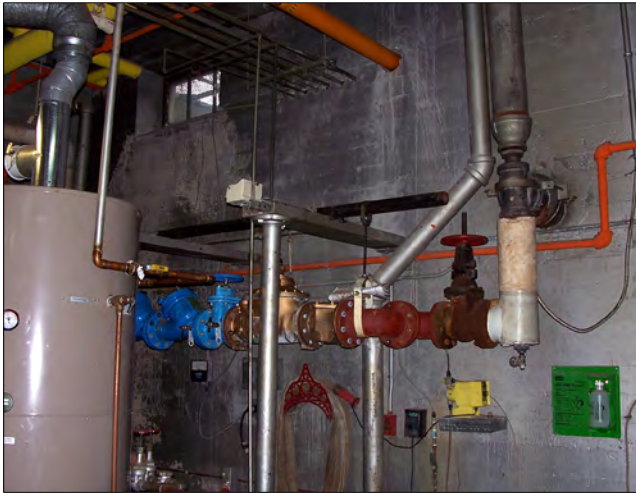
Water service entrance.
