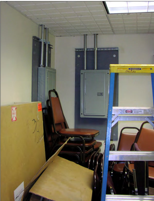
Access to electrical panels should not be blocked by stored items.
