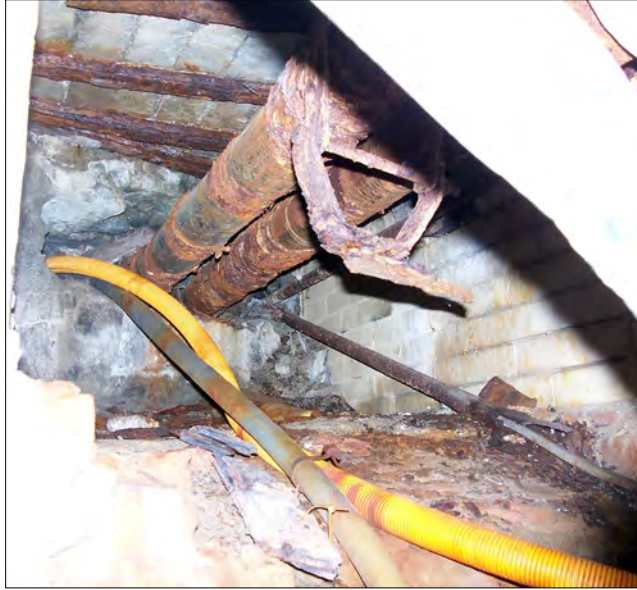
Deteriorating cooling tower piping in the service tunnel.
