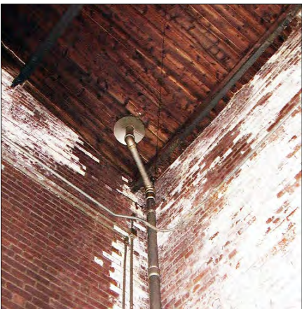
Efflorescence, the result of roof leaks, is visible on the brick walls of the drill shed above, and the gym shown below.
