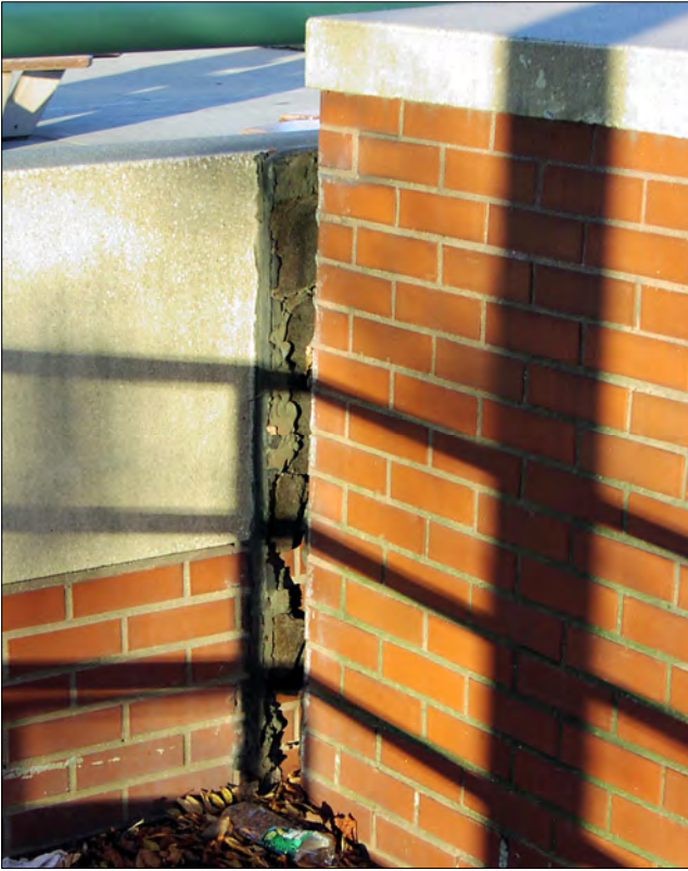
One of the site walls appears to have settled, resulting in cracks in brick mortar joints and separation from another site wall.
