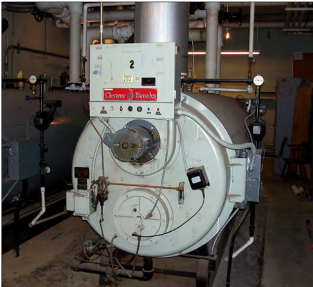
The old boiler in Harriman Hall should be replaced within the next ten years.
