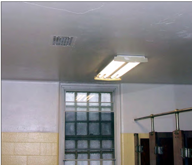
Gravity exhaust opening, located in some of the toilet rooms, would need to be replaced with exhaust fans.
