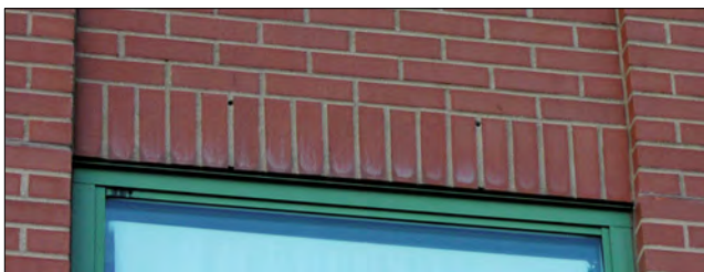
Interior water damage appears to be the result of improperly placed wall flashing and weep holes above windows.
