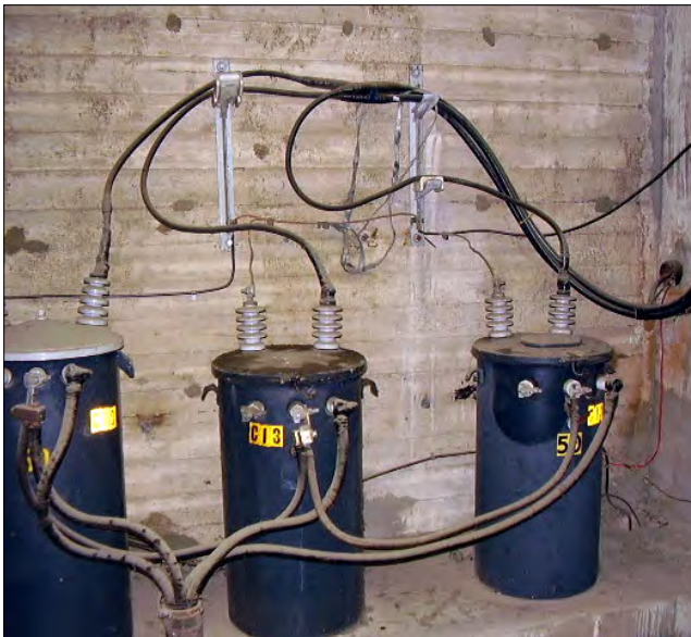
The building's transformers are old and in poor condition.
