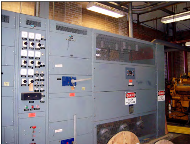
The main switchgear equipment and transformer in the Ice House are past their useful life and should be replaced.
