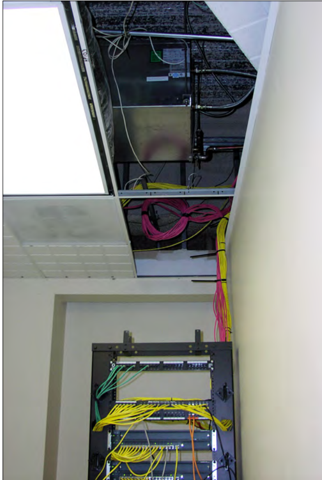
Water-source heat pumps are located above the suspended acoustic tile ceilings.
