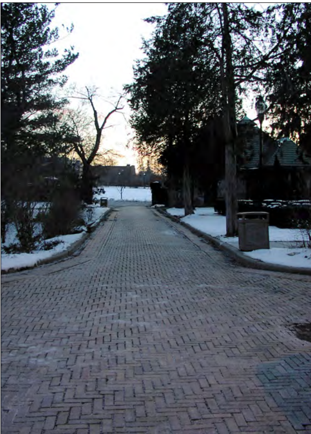
The paved road west of Horton Hall has settled above the utility tunnel that runs between Horton Hall and the Ice House. The pavers should be removed; the area should be regraded; and the pavers should be reinstalled.
