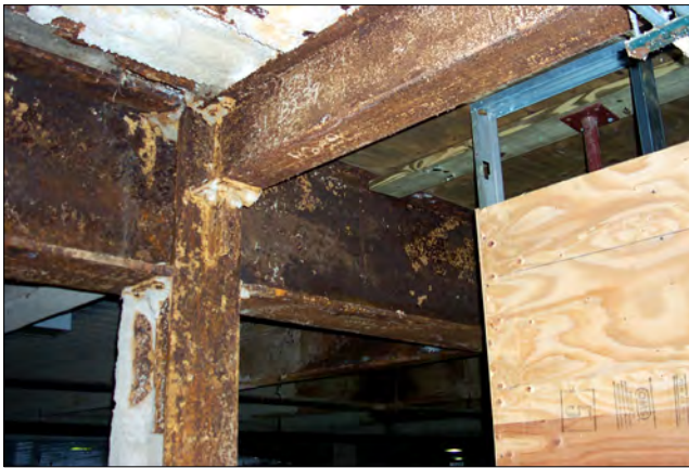
Water damage is evident in the parking garage beneath the Maple Building.
