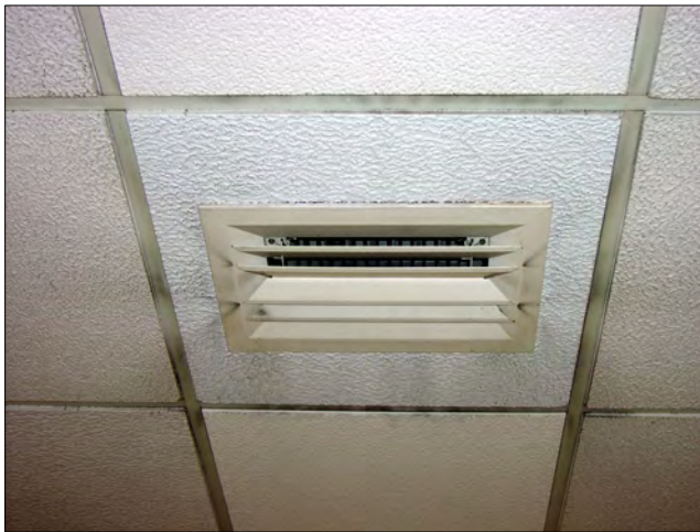
Black dirt can be seen at many air supply diffusers.
