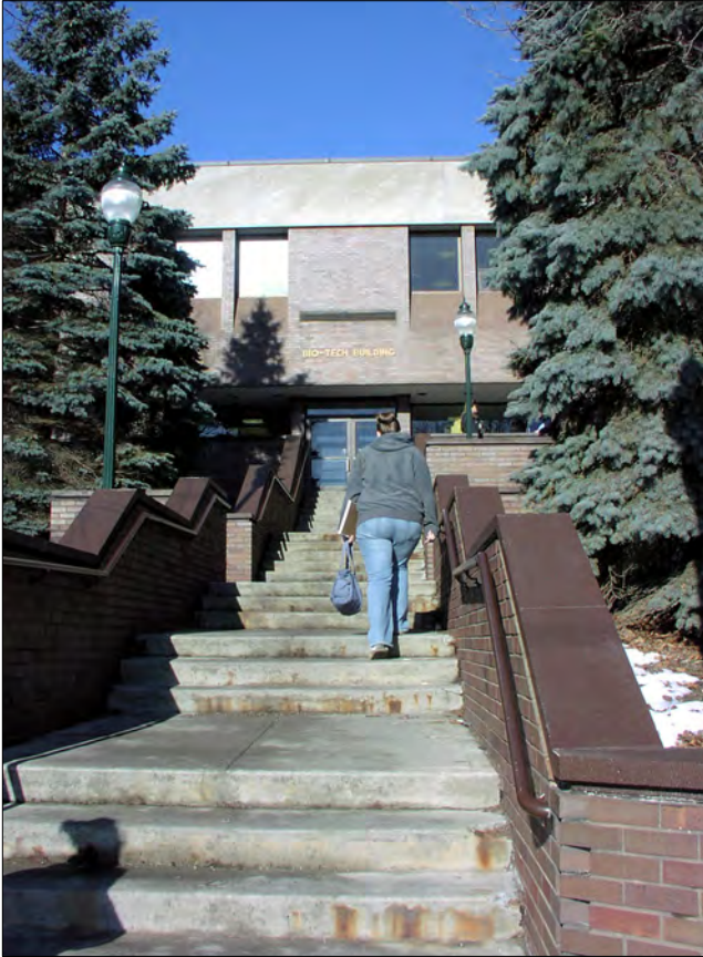
The exterior south stair to the Bio-Tech Building.
