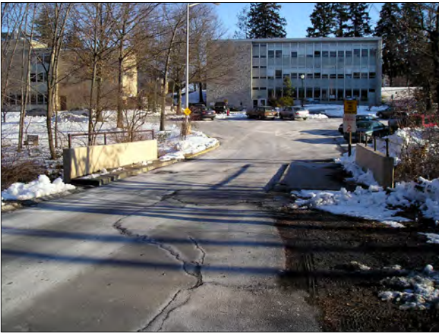
The College should consider widening the road and bridge at the entry to the Harriman Hall parking lot.
