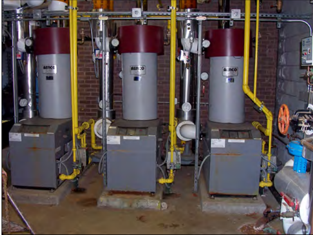
The boilers were recently replaced.
