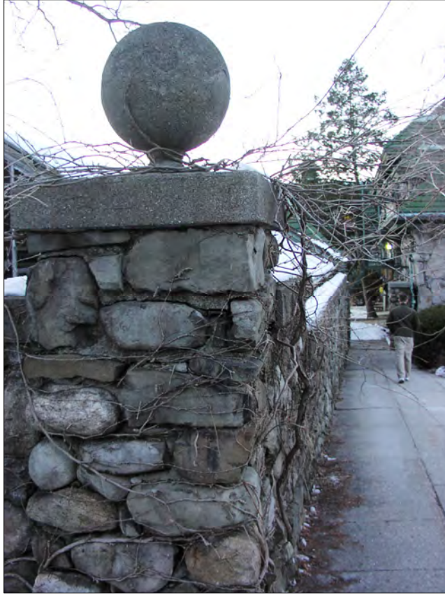
The stone site wall, a portion of which serves as the east wall of Greenhouse A, should be repointed.
