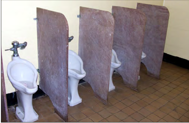
Existing toilet fixtures, including urinals, would need to be replaced with low flow fixtures.
