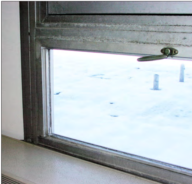
The building's windows are in poor condition and they are not energy-efficient. The College should replace the curtainwall system.
