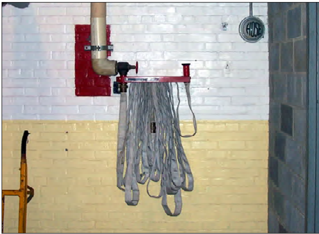
The building fire protection system consists of hose stations fed from the domestic water service.
