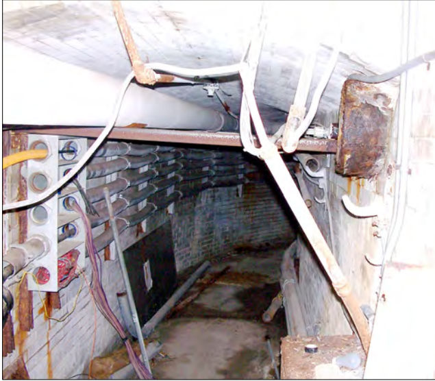
View of the underground service tunnel.
