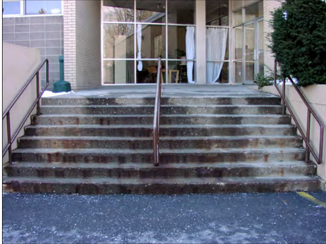
The exterior north stair is beginning to deteriorate and should be monitored.
