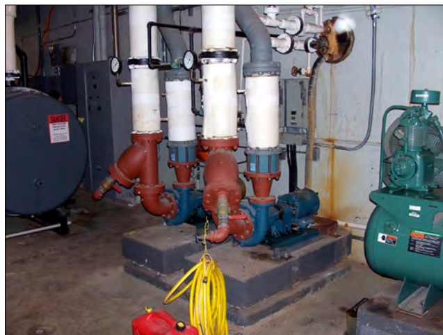
New control valves, dampers and suction diffusers should be installed.
