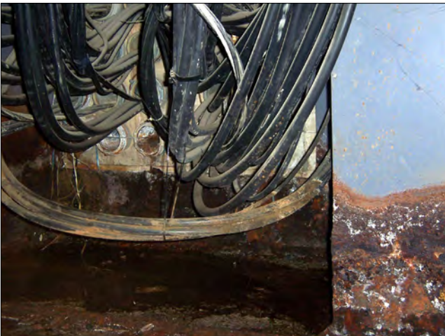
The electrical junction box in the basement of the Ice House is severely deteriorated because of water infiltration through the conduits.
