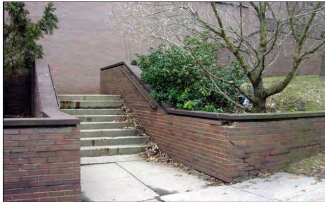
The site wall and stair at the southeast corner of the Bio-Technology Building are beginning to deteriorate.
