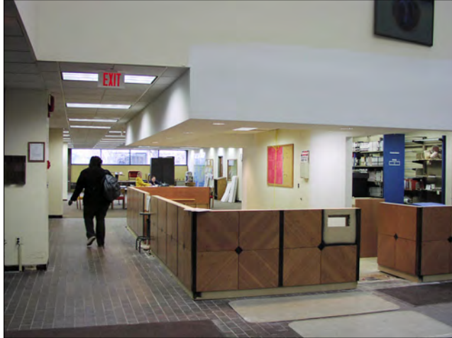
The new circulation counter, under construction.
