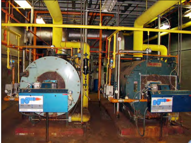
The two fire-tube boilers would need to be replaced if the building was to remain in use.
