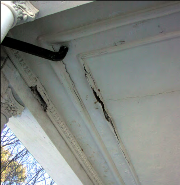
Damage to flat roof sections has affected the ceilings below.
