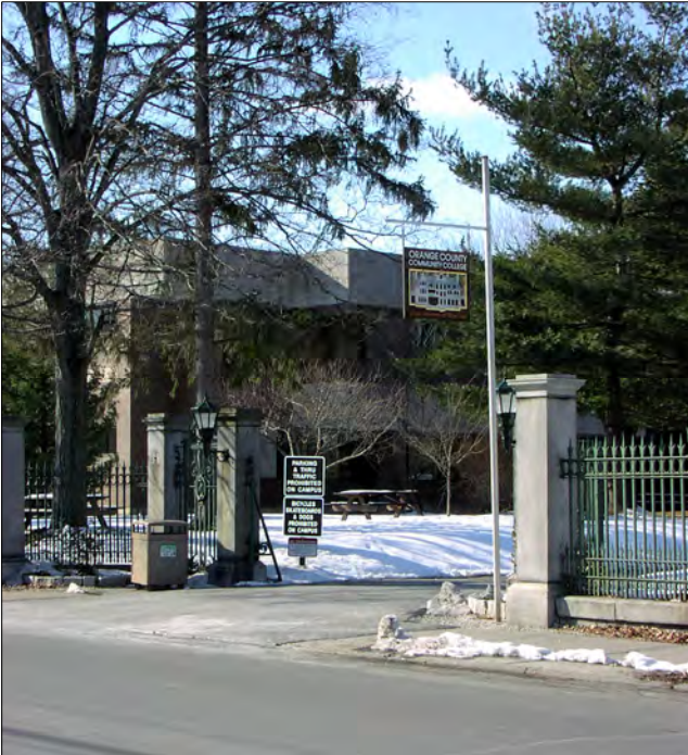
The main entry to the campus core is used by both vehicles and pedestrians.
