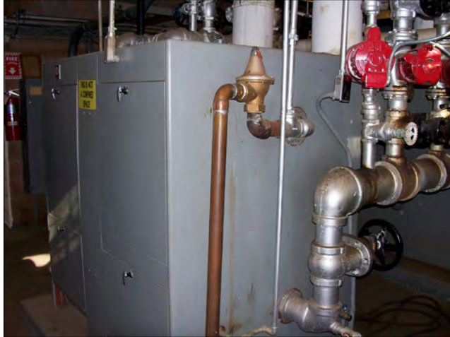
The two old boilers should be replaced.
