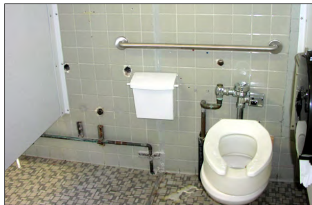
Modifications to the toilet rooms have made them more accessible, but aesthetic improvements are still needed.
