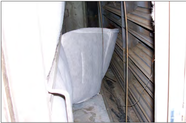
A displaced filter on an air-handling unit should be put back in place to improve indoor air quality in the Commons.
