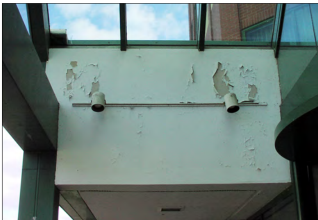
Exterior soffits need to be repainted.
