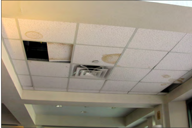
Damaged ceiling tiles should be replaced.
