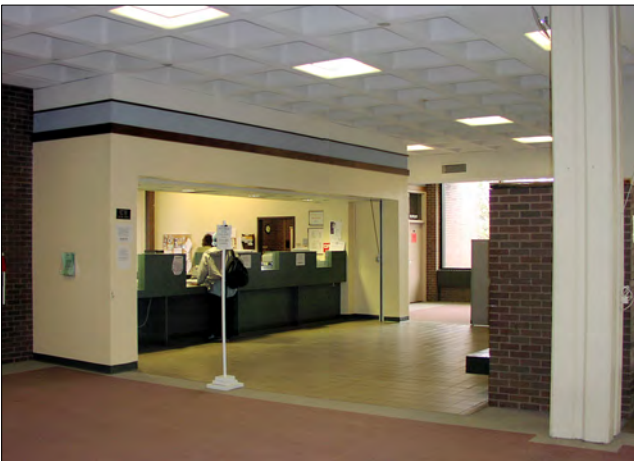
A roll-down fire shutter was installed at the Bursar's counter, located in the main lounge on the second floor.
