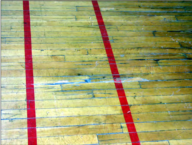
The gymnasium floor is in poor condition. It should be replaced and new bleachers and partitions should be installed.
