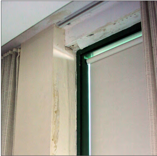
Interior water damage appears to be the result of improperly placed wall flashing and weep holes above windows.
