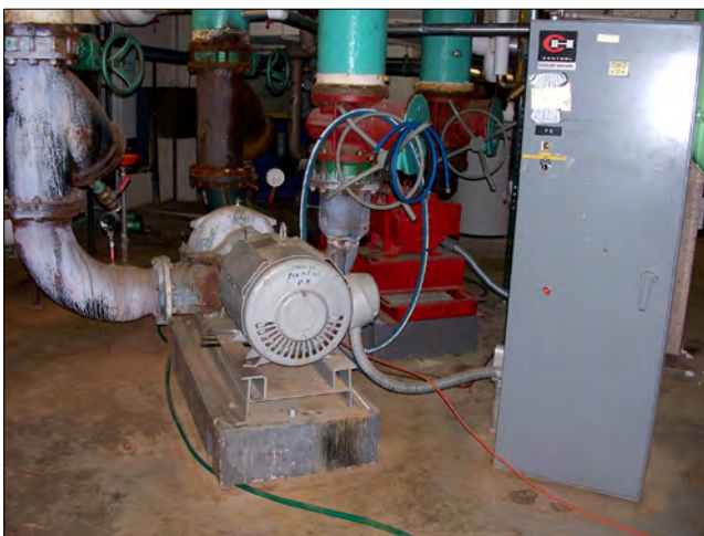
The existing tower pumps should be replaced.
