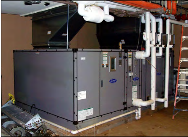
New air-handling unit located in the basement.
