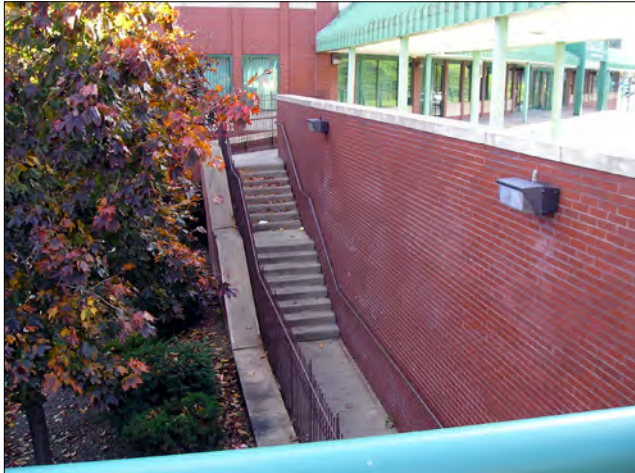
The site stair between the Key Bank and Maple Buildings collects wind-blown trash and leaves and is difficult to maintain.
