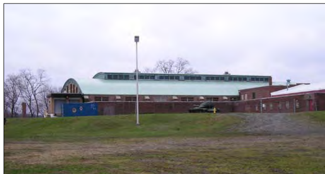
The barrel-vaulted drill shed has an interesting structure, but the configuration of the building does not lend itself to conversion for college use.
