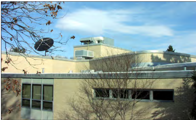
Roof-top air-conditioning equipment can be seen on the roof of Orange Hall.
