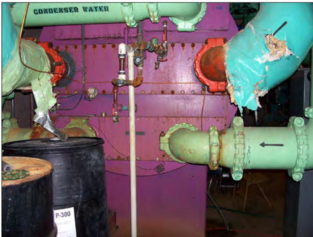
The existing absorption chiller is being replaced.
