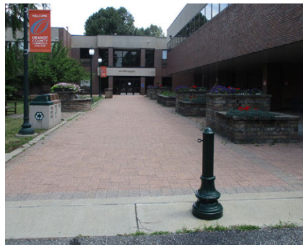
Failing Planters & Inconsistent Furnishings
