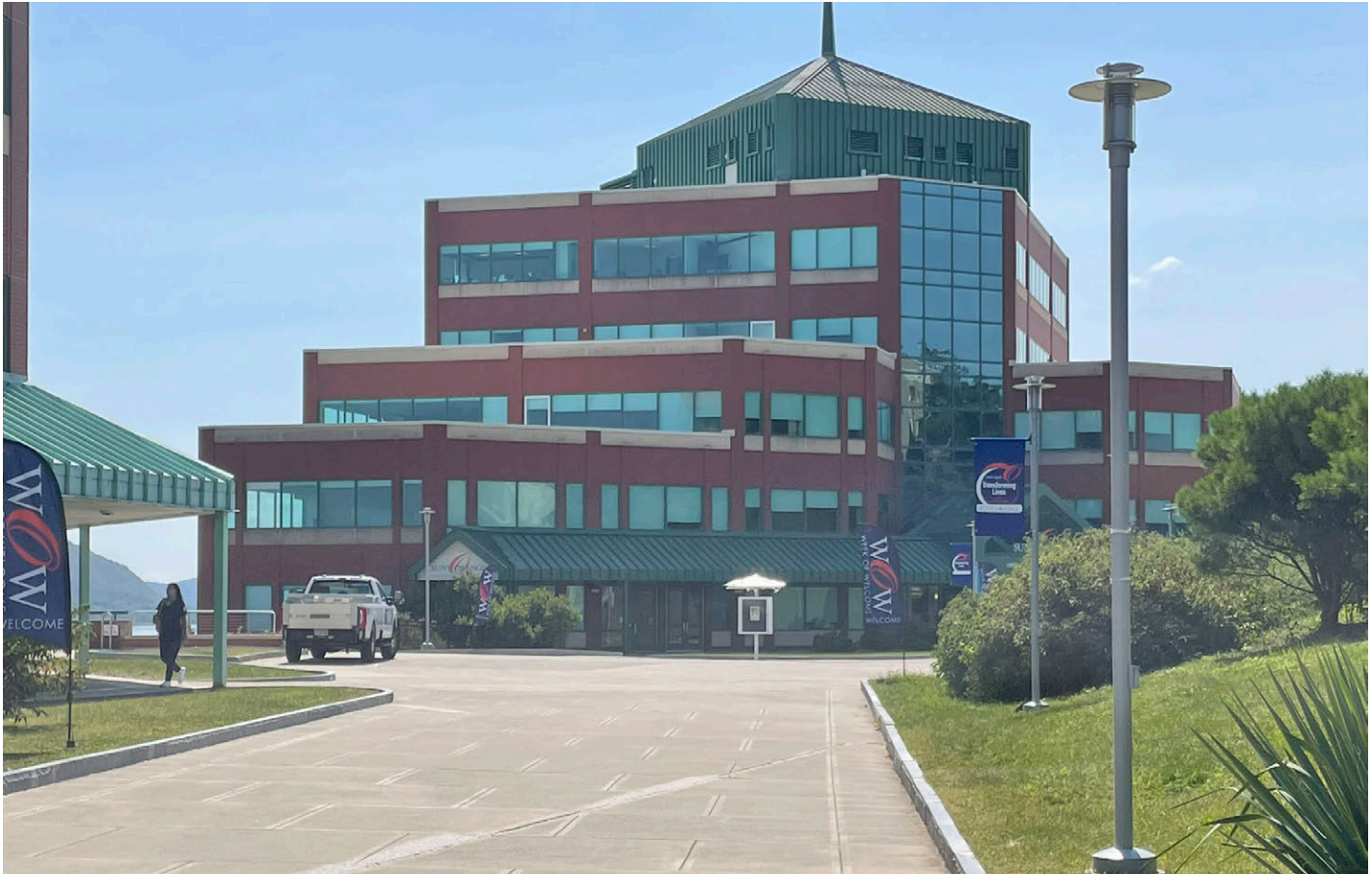
Existing Pedestrian Plaza
