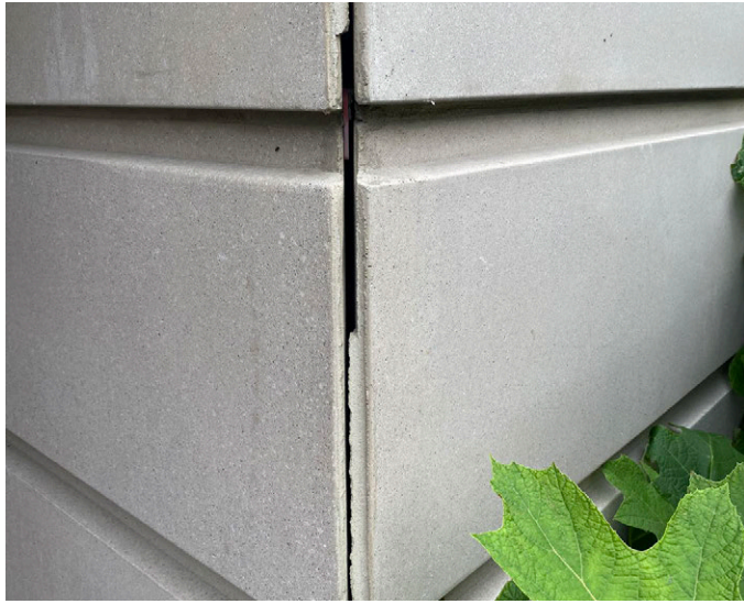
Missing Sealant
