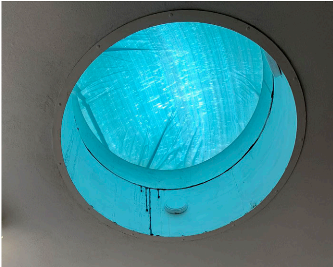
Leaking Skylight
