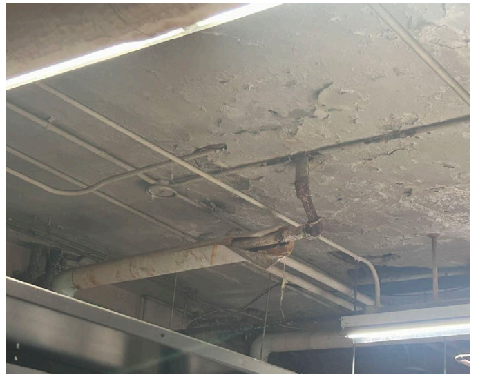
Deteriorated Piping
