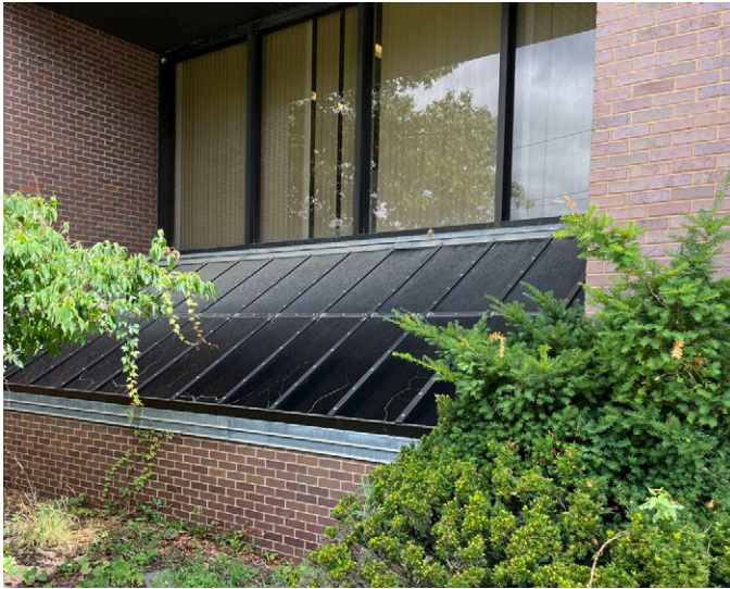
Original Window System in Fair Condition
