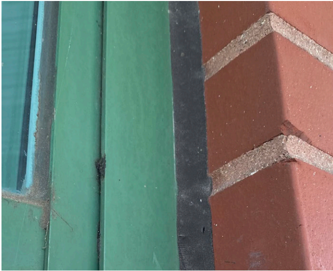
Failed Sealant
