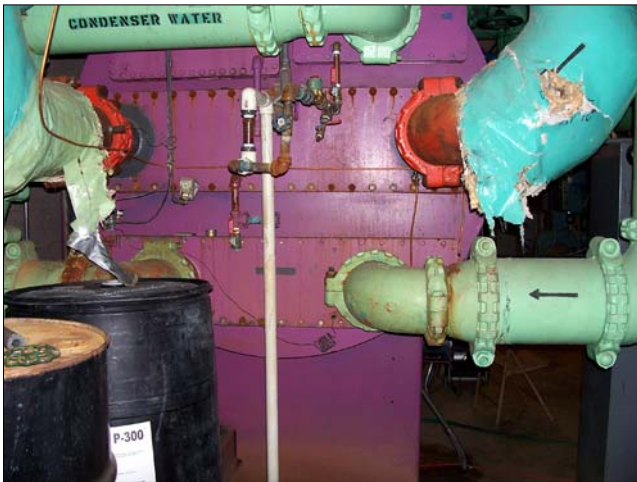
The existing absorption chiller is being replaced.
