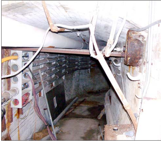
View of the underground service tunnel.
