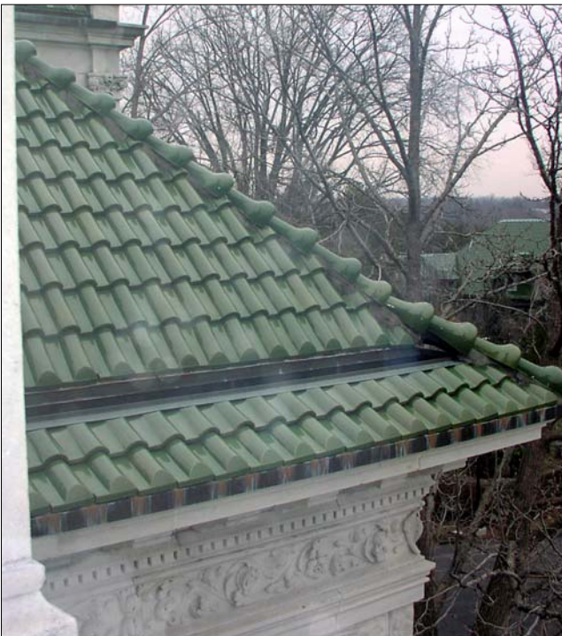
Gutters originally used steam to help melt snow and ice on the roof. This system was not duplicated when the new clay roof was installed.
