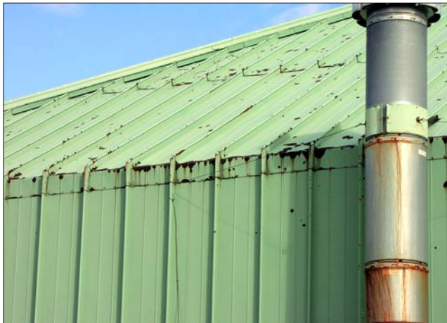
A new ballasted membrane room system will be needed and the standing-seam metal roof needs repairs.
