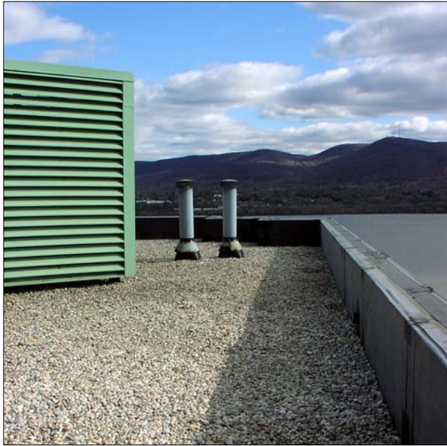
A new ballasted membrane room system will be needed and the standing-seam metal roof needs repairs.
