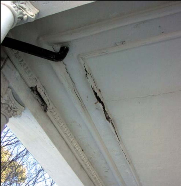
Damage to flat roof sections has affected the ceilings below.
