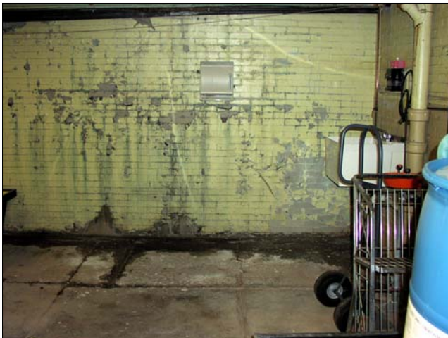
Water can be seen seeping into the basement of Horton Hall at the base of the service tunnel door, shown above. Water infiltration also occurs at the base of the basement wall, as shown below.
