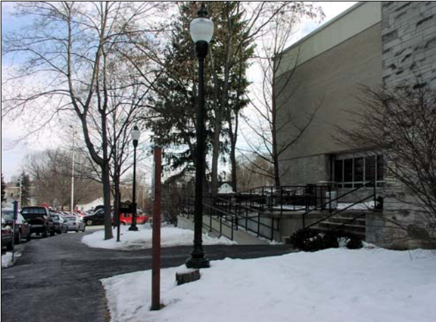
A new concrete accessibility ramp was installed at the south entrance of the building. A new site stair (below) was constructed on the west side of the building.
