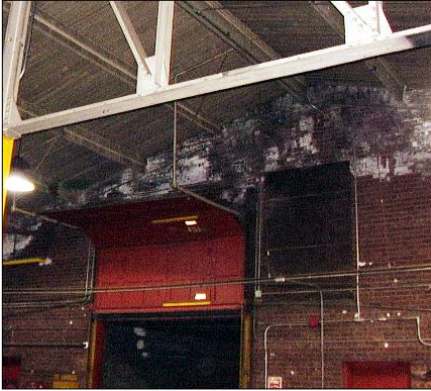
Efflorescence, the result of roof leaks, is visible on the brick walls of the drill shed above, and the gym shown below.
