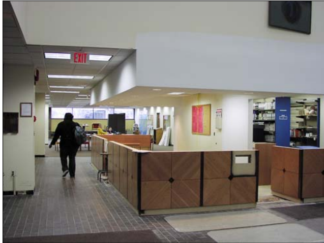
The new circulation counter, under construction.
