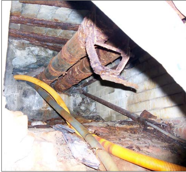
Deteriorating cooling tower piping in the service tunnel.
