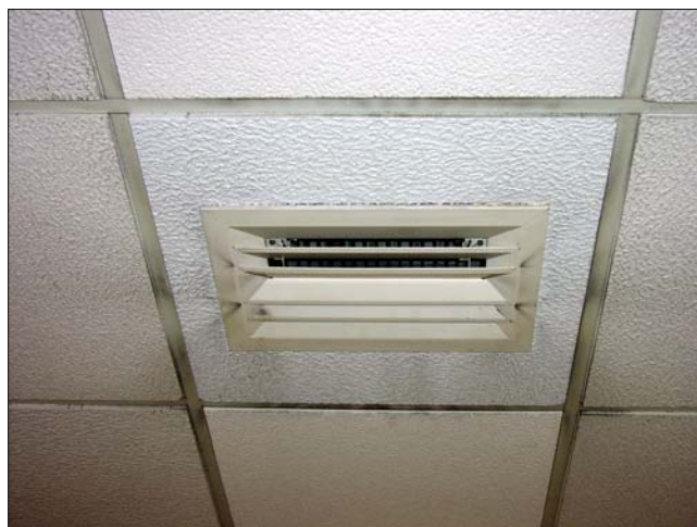
Black dirt can be seen at many air supply diffusers.
