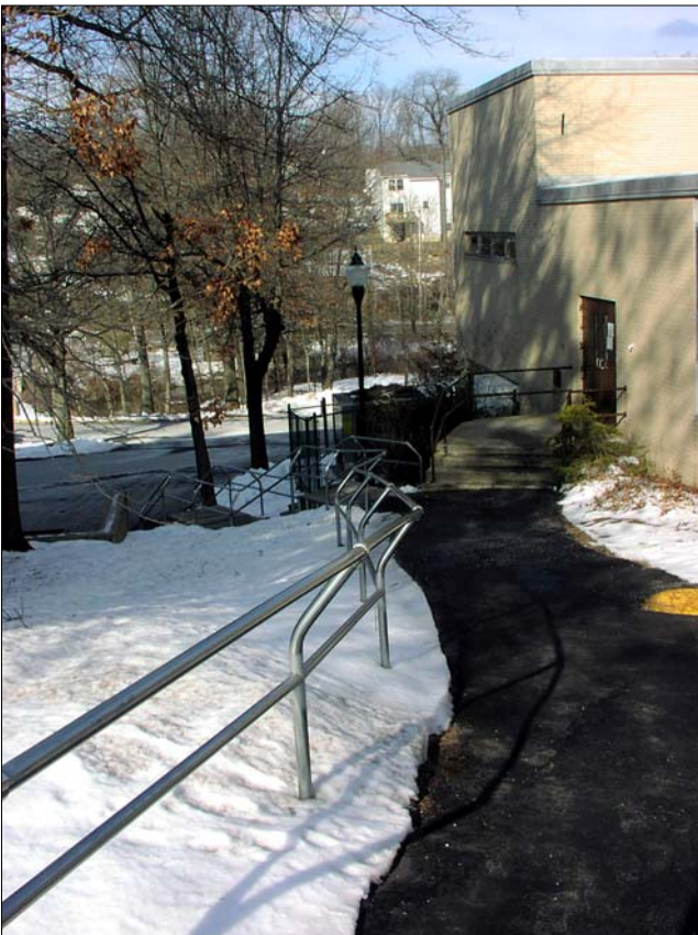
A new concrete accessibility ramp was installed at the south entrance of the building. A new site stair (below) was constructed on the west side of the building.
