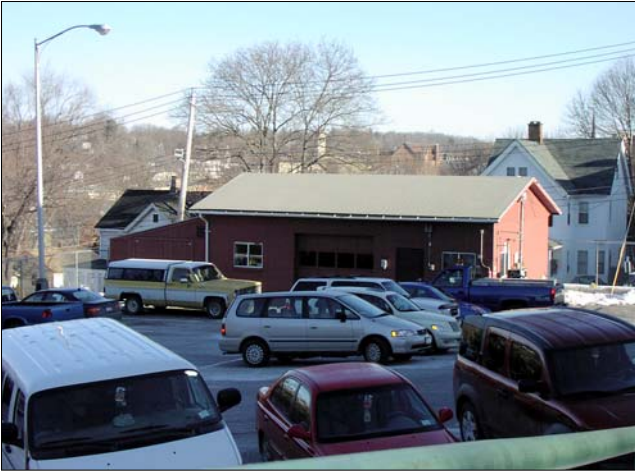
The HVAC Shop sits behind Horton Hall.
