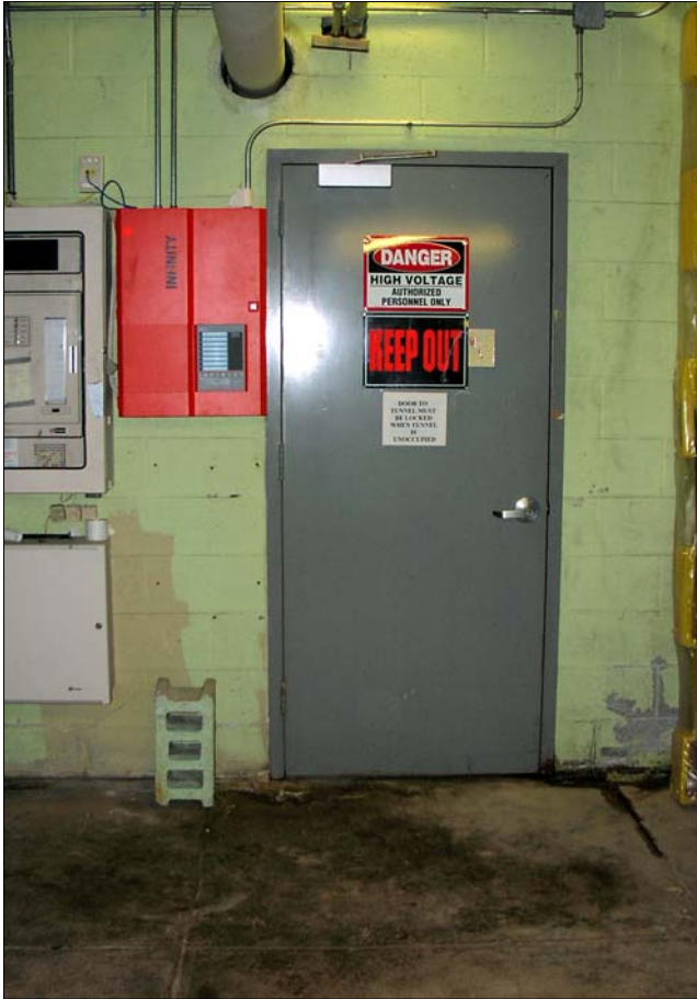
Water can be seen seeping into the basement of Horton Hall at the base of the service tunnel door, shown above. Water infiltration also occurs at the base of the basement wall, as shown below.
